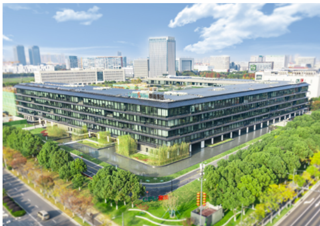
Rooftop and overhang PV installations
