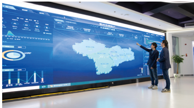
The smart integrated energy management platform clearly presents corporate energy consumption data
