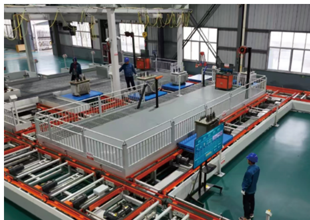
The first green dismantling line for waste transformers independently developed by State Grid Dezhou
