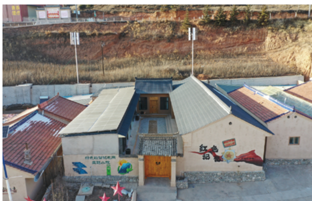
Building an all-electric zero-carbon green energy courtyard – Revolutionary Liupan Mountain Green Energy Courtyard
