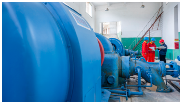
Power company employees conduct a safety inspection at the Junyang Hydropower Station in Dajun Town to ensure safe and stable operations
